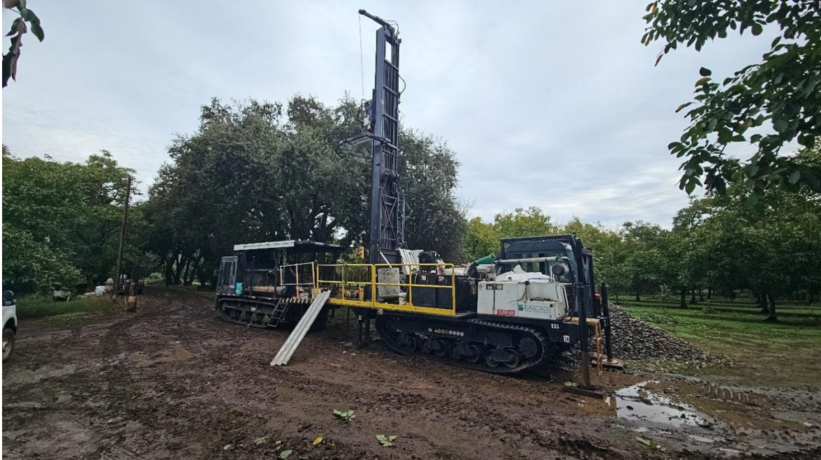
Photograph 3. Sonic drill rig used for completion of soil borings.
