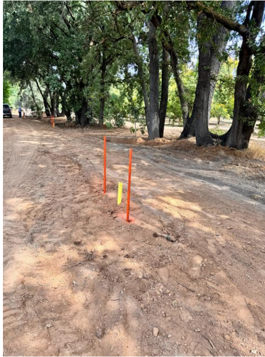
Photograph 10. Observation points (yellow pipes) installed within trench to record water levels during pilot testing.
