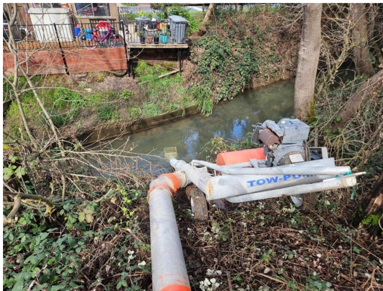
Photograph 14. Pump intake going into Comanche Creek.
