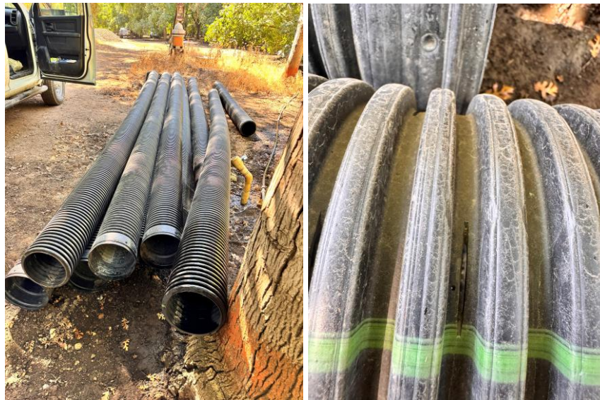
Photograph 9. Eight-inch perforated pipe installed in bottom of trench. Photograph on right shows perforation.
