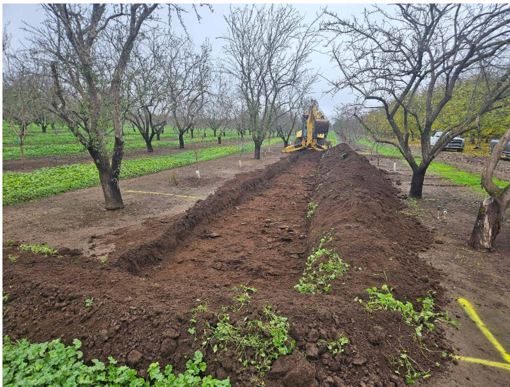
Photograph 18. Construction of South infiltration basin.
