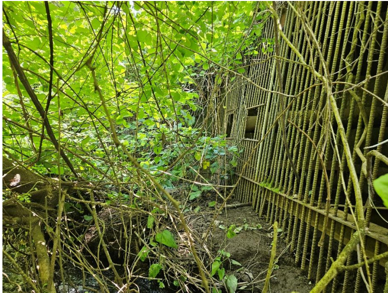
Photograph 20. Photograph of old diversion structure looking from Comanche Creek.
