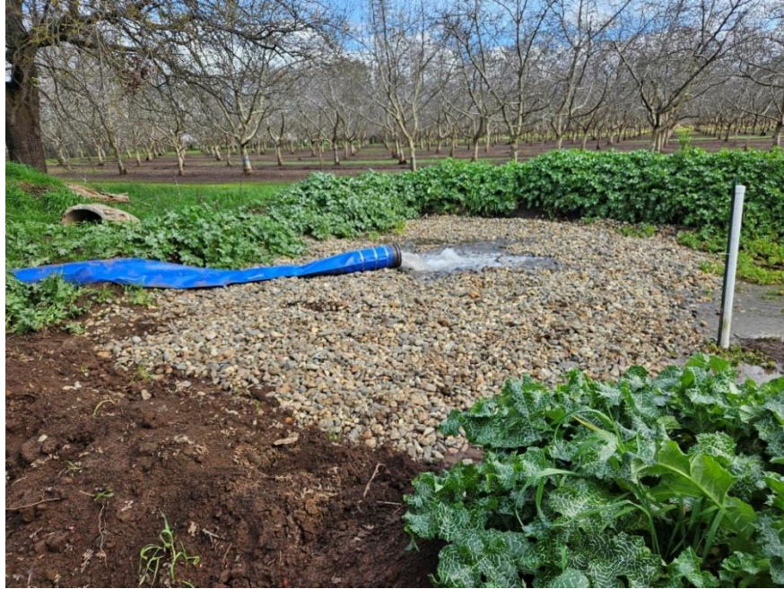
Photograph 15. Discharge line from Comanche Creek going into north end of infiltration basin.
