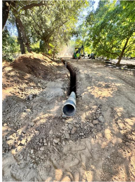
Photograph 8. Photograph showing excavation of trench with perforated pipe installed.
