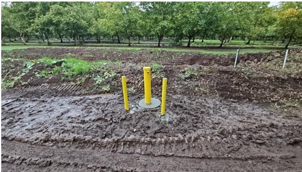
Photograph 5. Surface completion of monitoring well as Site S1
