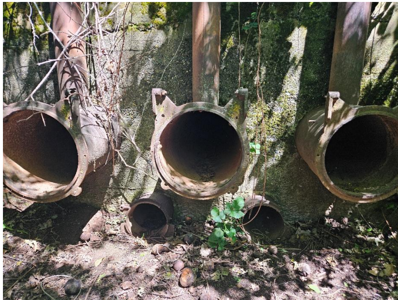
Photograph 21. Picture of old diversion structure looking from Site S1.
